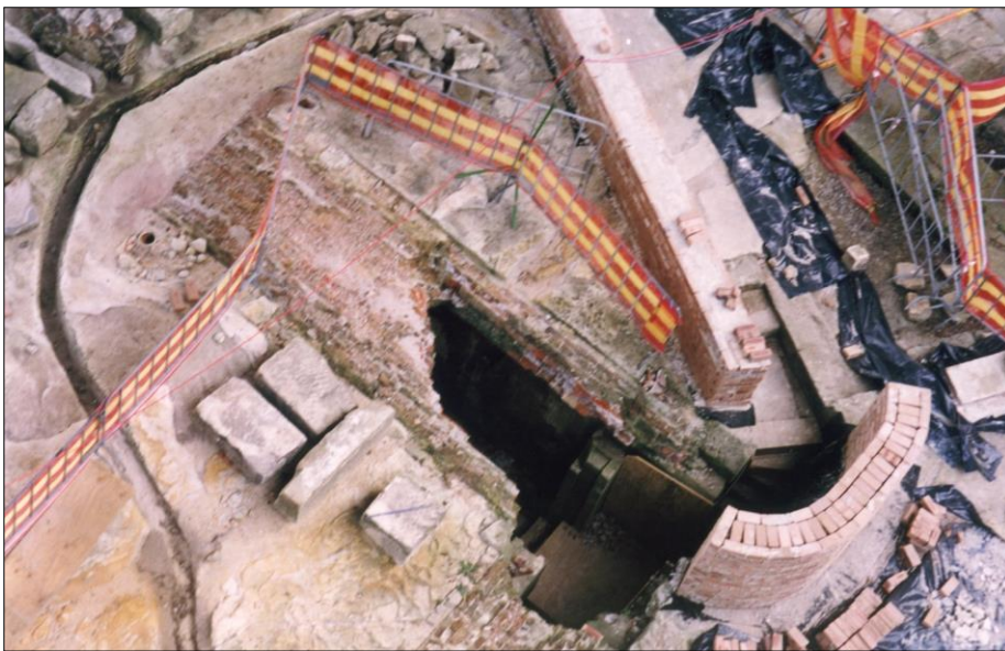
Small powder magazine under restoration, Dawes Point Battery 2001
